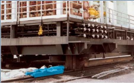
Gripper Jack in a construction yard used to position modules, structures, and equipment.
