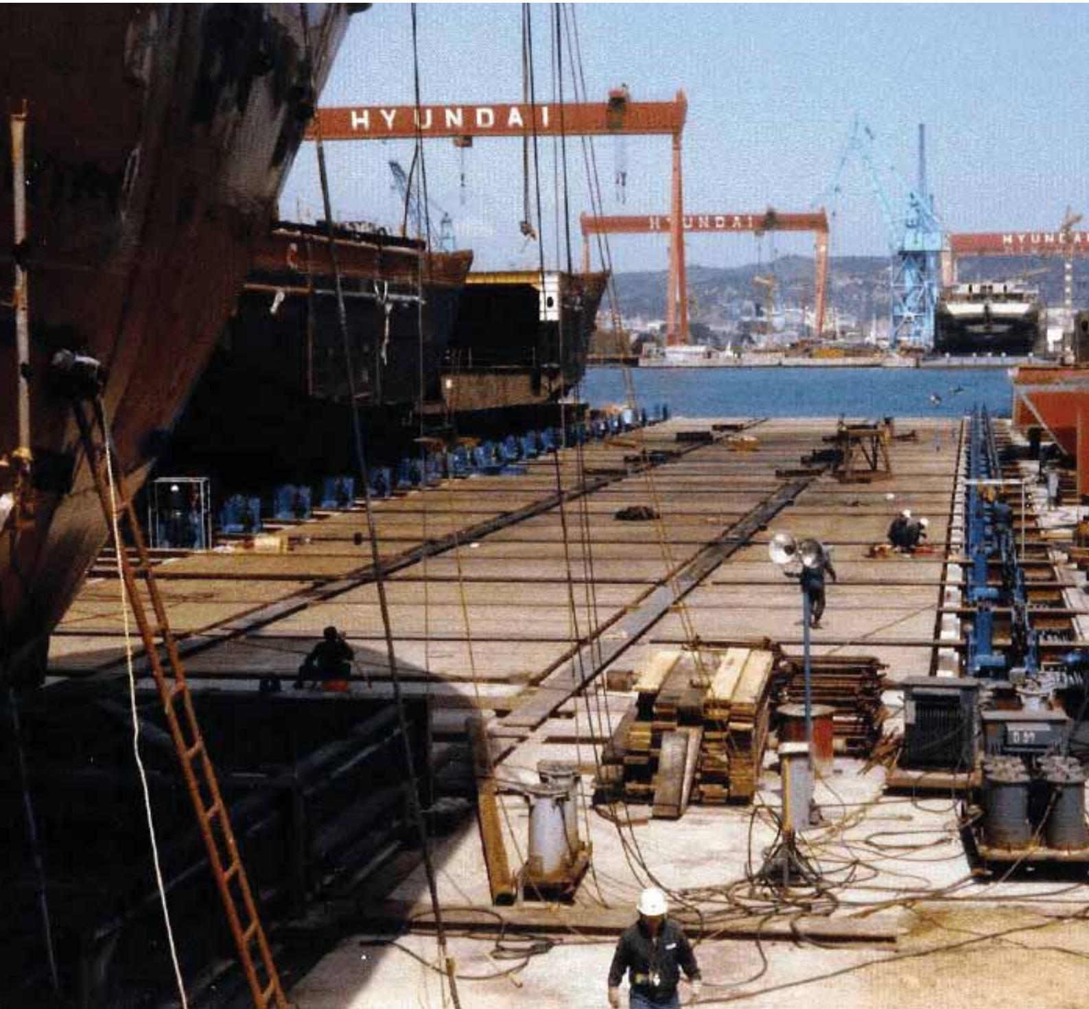
A 4,200 tonne capacity Bardex shiplift with side and longitudinal transfer system
