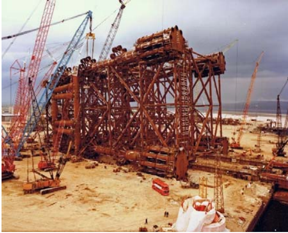
Figure 3 A low volume skidding system used for jacket loadout.
